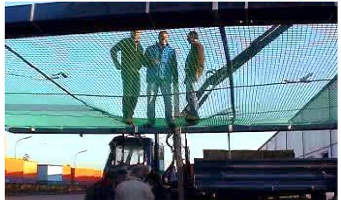
Figure 13. Work Platform Net (Photograph courtesy of Dr. M. Einhaus).
