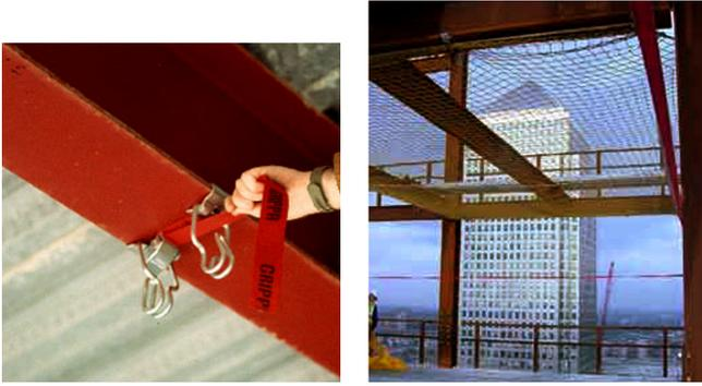
Figure 9. Safety Net in Construction (Photograph courtesy of SFP Inc.).
