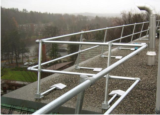
Figure 5. Example of Permanent Non-holes-in-roof Guardrail (Photograph courtesy of KeeGuard Company).
