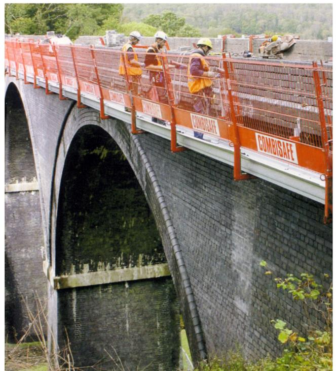
Figure 4. Example of a Temporary Guardrail (Photograph courtesy of Combisafe Company).
