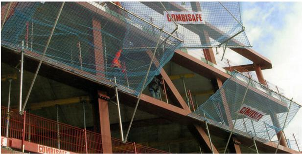
Figure 10. Safety Net in Construction (Photograph courtesy of Combisafe Company).
