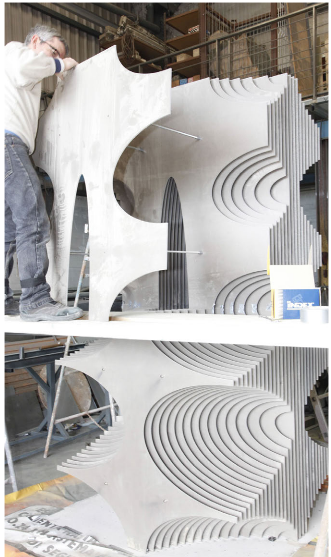
Figure 14. Assembly and post-tensioning of tile sheets (Photo: Jordi Font de Mora, Grupo on Market).
