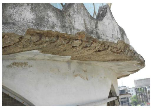
Figure 4. Reinforcement Completely Exposed to External Environment in Dome C.
