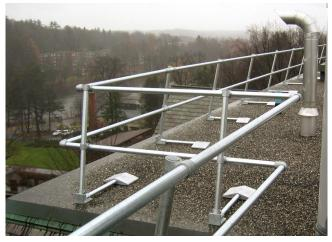
Figure 5. Example of Permanent Non-holes-in-roof Guardrail (Photograph courtesy of KeeGuard Company).
