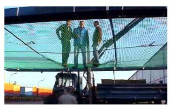
Figure 13. Work Platform Net (Photograph courtesy of Dr. M. Einhaus).
