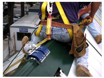
Figure 8. Example of FAS attached to permanent Horizontal Lifeline (Photograph courtesy of Saferidge Safety System Company).
