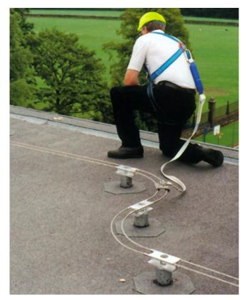
Figure 15. Permanent Horizontal Lifeline (Photograph courtesy of Tractel Inc.).
