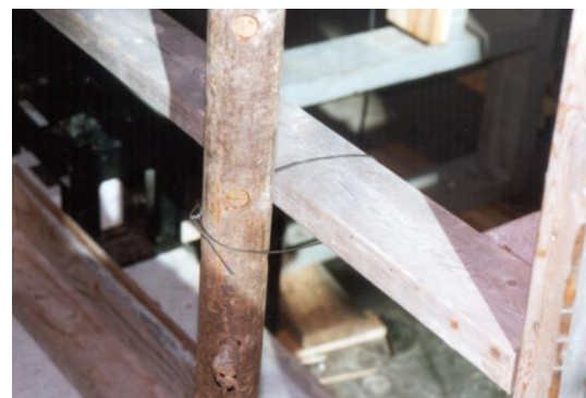
Figure 7. Wooden guardrail attached to shoring jacks with # 16 binding wire - Overlapping of guardrails on a shoring jack.
