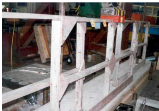
Figure 7. Wooden guardrail attached to shoring jacks with # 16 binding wire - Overlapping of guardrails on a shoring jack.
