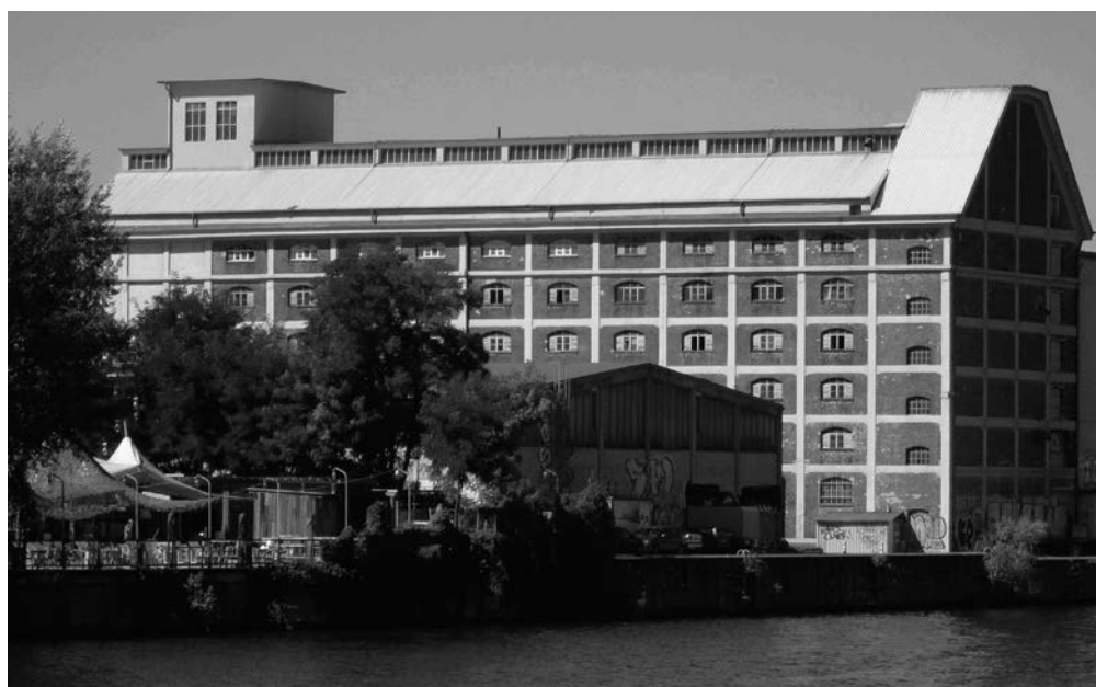
Figure 3. North-east facade (axis I) of the Victoria Warehouse showing the frame structure of the floor storage on the right, 2016.
