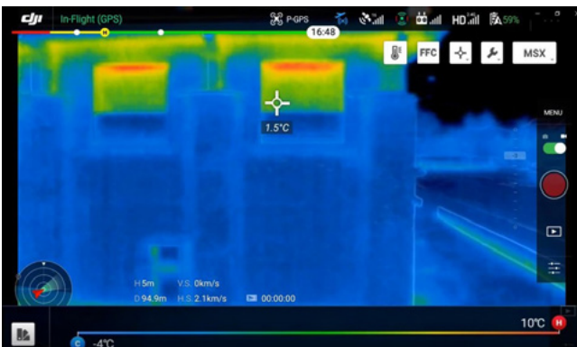
Figure 8. Temperature differences detected by the thermal camera: Windows and door.
