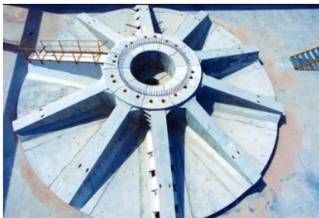
Figure 5. Picture of the Artepref precast foundation prototype (Artepref).
