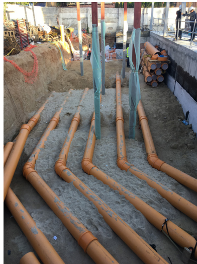
Figures 8. Visualization of the installation through a porthole, visualization of the Canadian wells and insulation on the façade.
