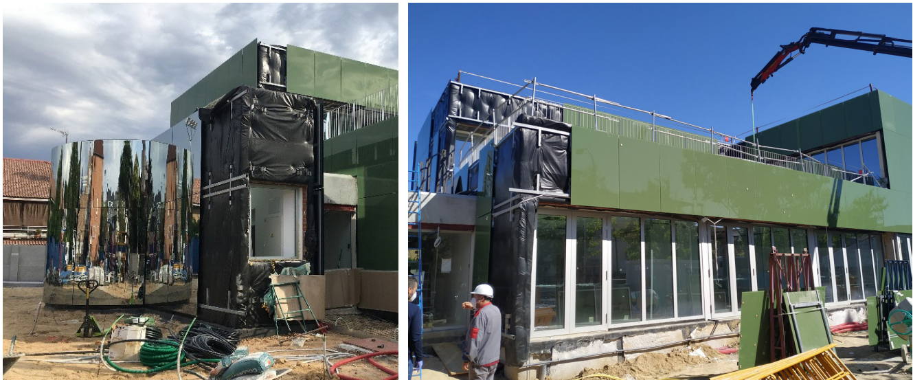
Figures 14. Construction of the BRAINS school. Placement of curved mirrors and glass in the envelope.
