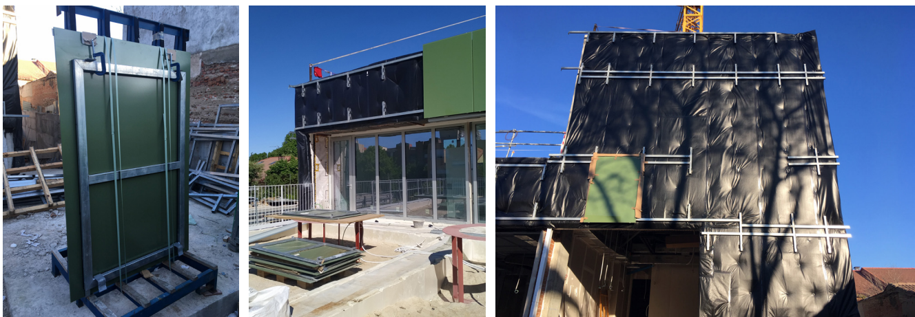
Figures 2. Large thicknesses of continuous thermal insulation throughout the building skin. Carpentry with tripalut glass.
