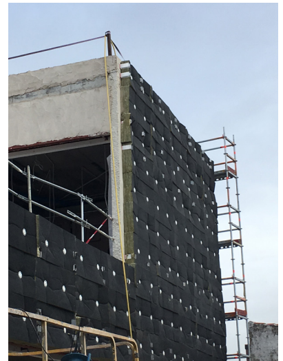
Figures 8. Visualization of the installation through a porthole, visualization of the Canadian wells and insulation on the façade.
