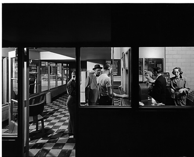
Figura 6. Downtown Parking Garage , 1953, Pittsburgh. Fotografía de Harold Corsini. (Cortesía de Carnegie Museum of Art. Collection of Photographs, 1894-1058.)
