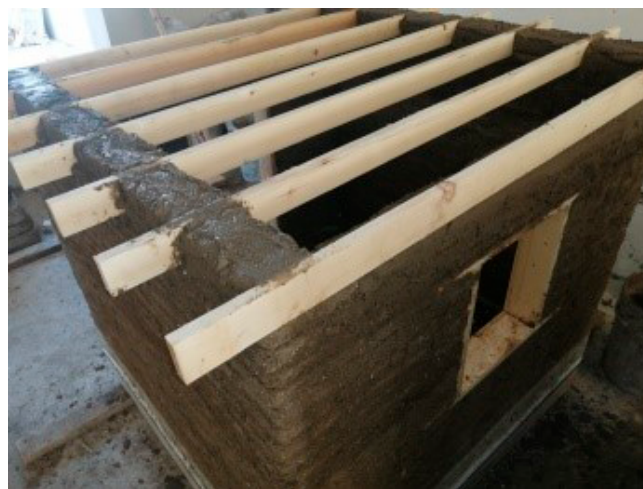
Figure 5. Roof beams and framing in spans
