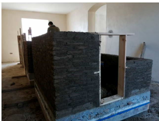
Figure 4. Foundation and wall construction
