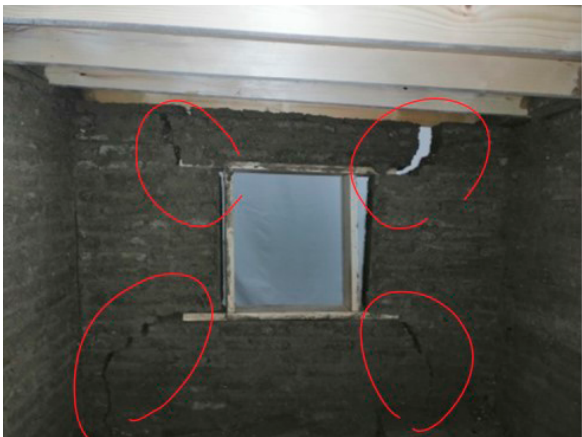
b. Large racks around the window opening, interior view
