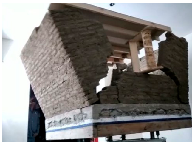
b. Total collapse, side backside view.
