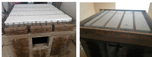
a. Roof slab for H-2 specimen b. Roof slab for H-3 specimen Figure 10. Construction process of H-2 and H-3 specimen roof slab
