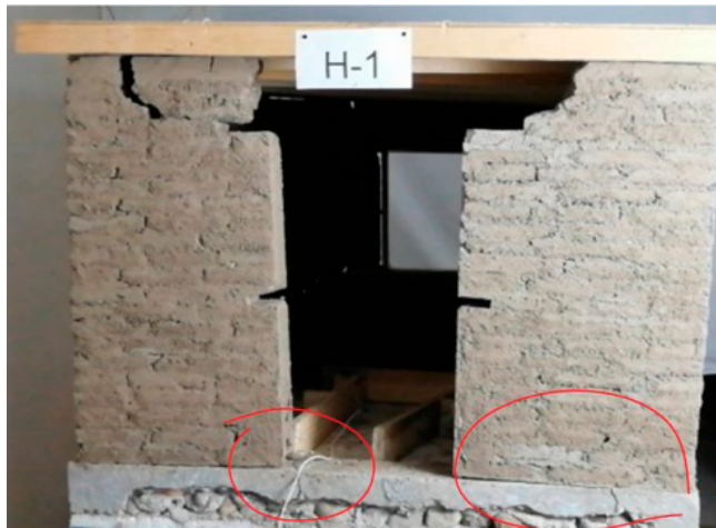
a. Extreme door damage and foundation fracture, front view
