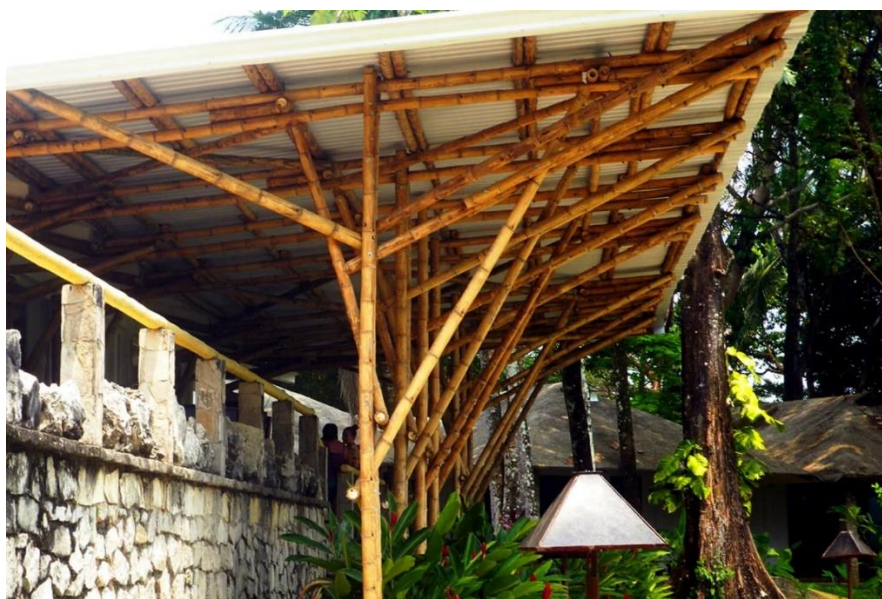
Figure 4. Cantilever of the extension
